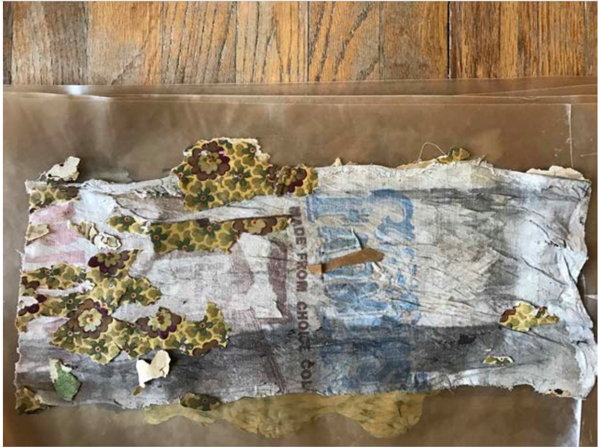
7. Seventh layer of wallpaper in Addition Room 4.
