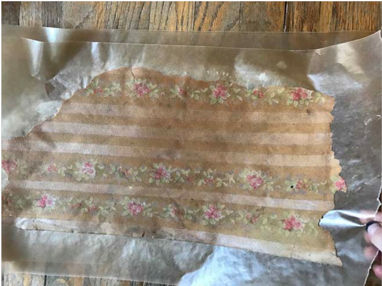
3. Third layer of wallpaper in Addition Room 4.
