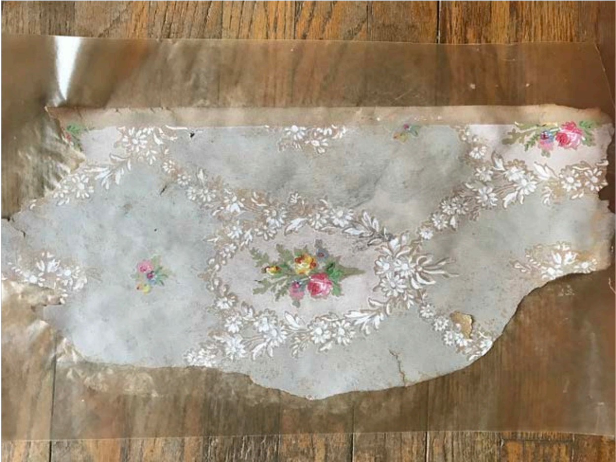
1. Top Layer of Wallpaper, currently visible on the walls of the interior of Addition Room 4.
