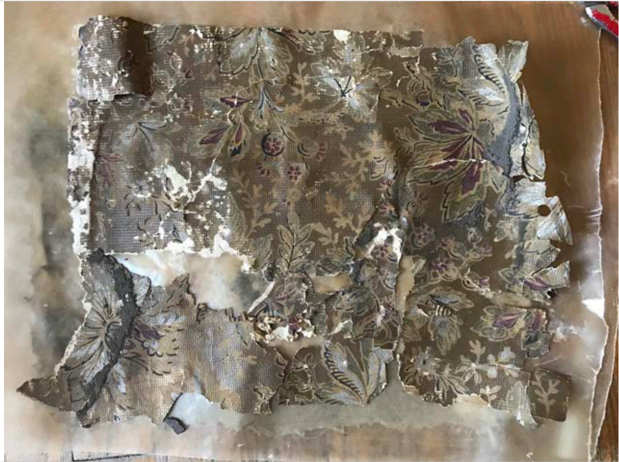
5. Fifth (oldest) layer of wallpaper in the Victorian Back Room.
