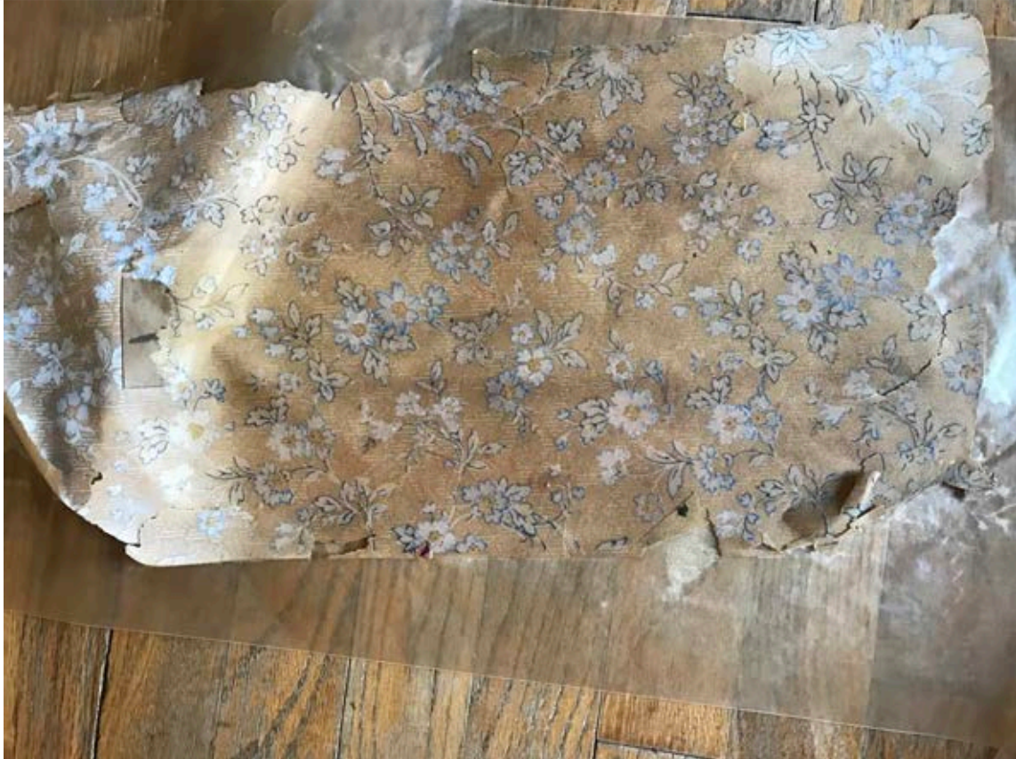
1. Top Layer of Wallpaper, currently visible on the walls of the interior of Addition Room 5.
