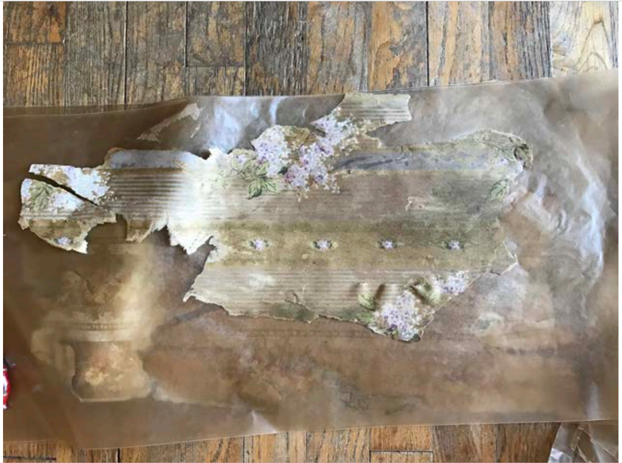
3. Third layer of wallpaper in Addition Room 5.
