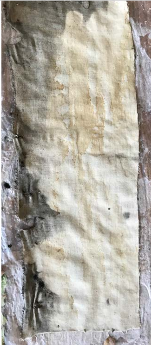
3. Linen backing, surface wallpaper is attached to.
